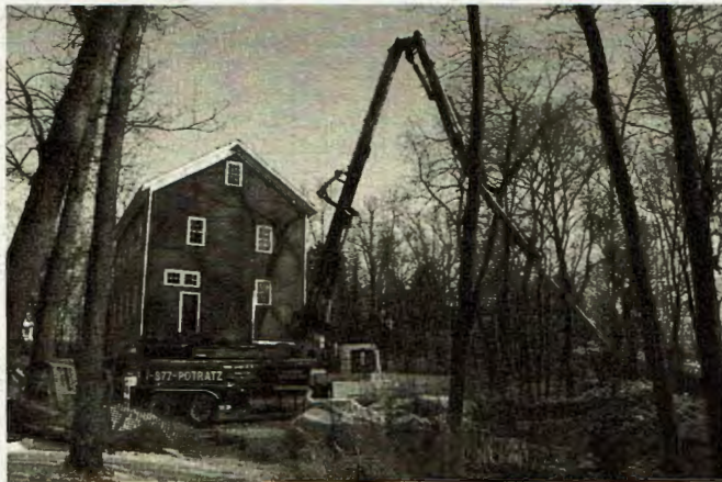
Work on the Mill Foundation
